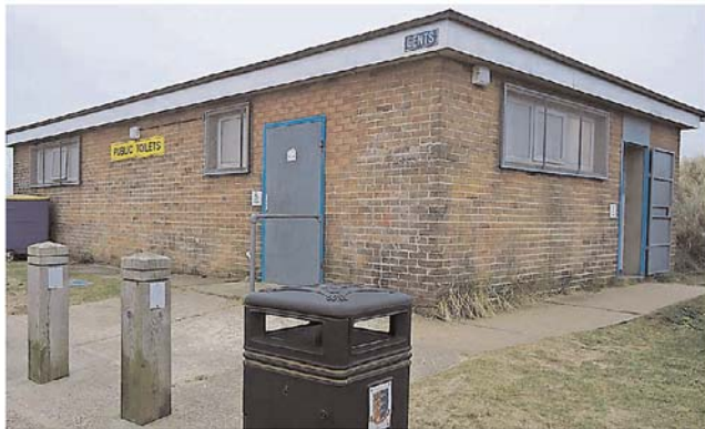
■ Winterton on Sea's public toilet, which is set to close.
